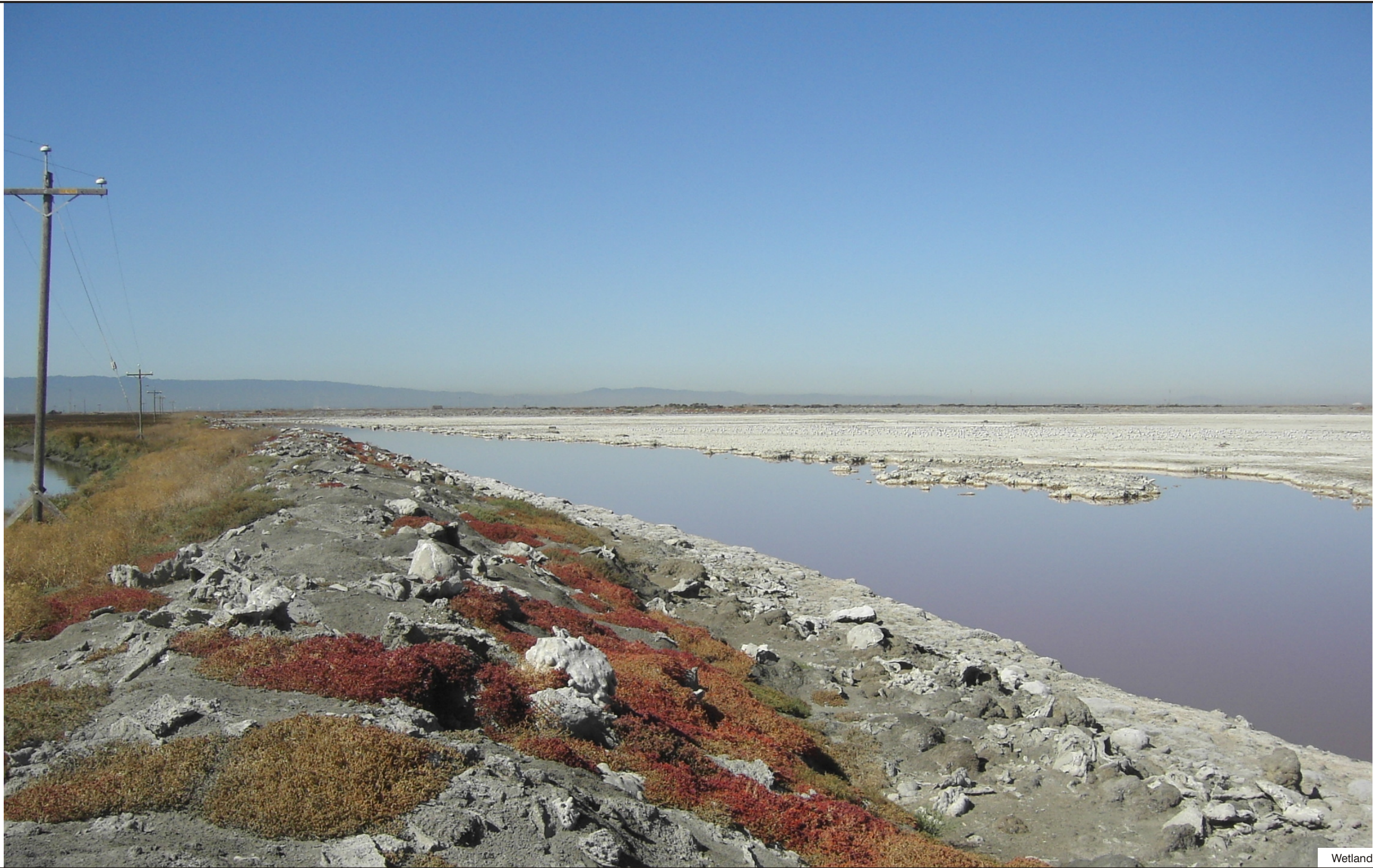
Photo from atop Pond A19 levee, October 10, 2005. Note gypsum blocks on levee surface, from excavating borrow ditch materials during levee maintenance. Note gypsum-covered pond surface. Note borrow ditch between levee and pond surface. Coyote Creek on left.
